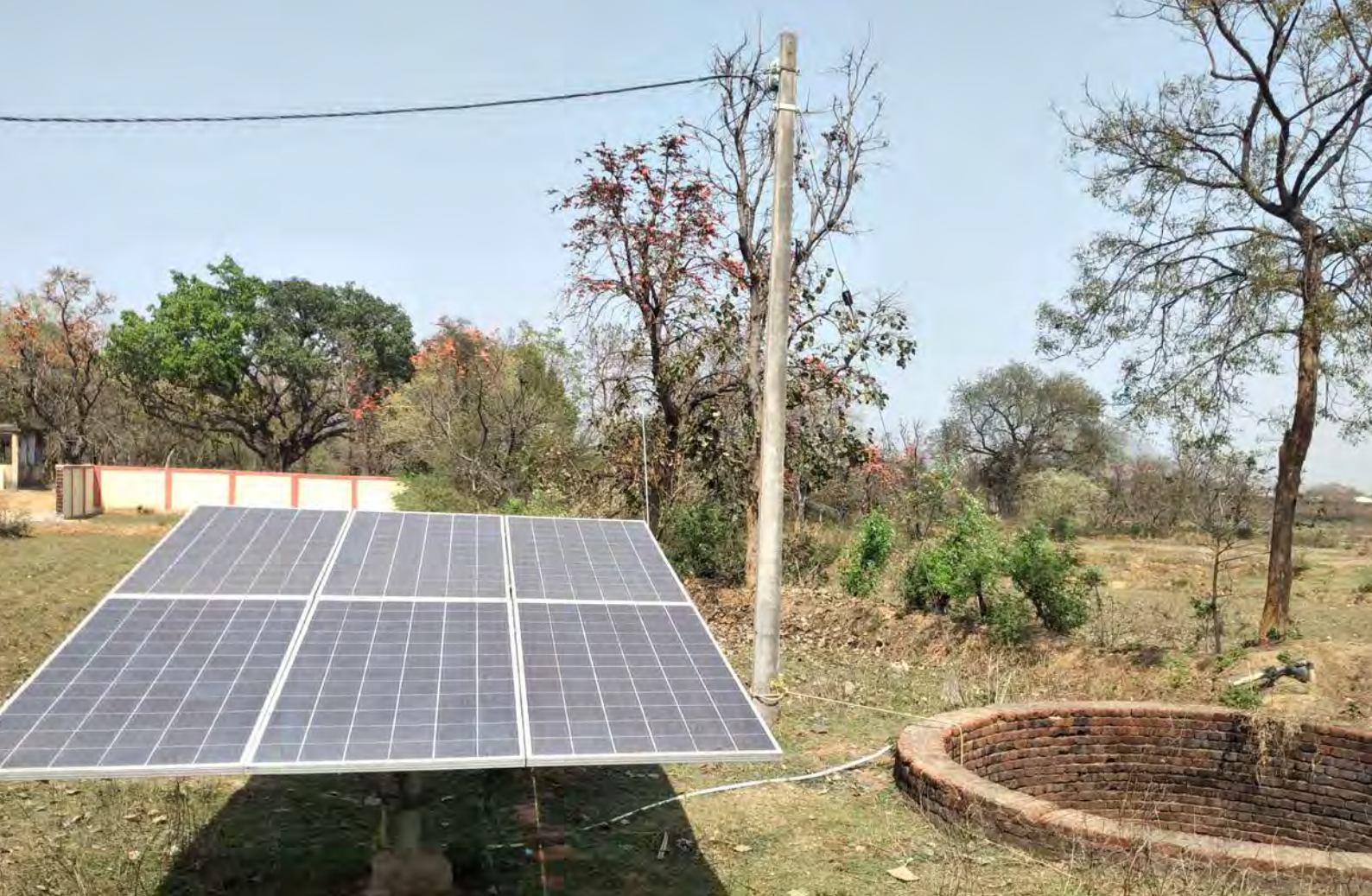
Solarized Agri irrigation system through surface pumping, Dhanbad
